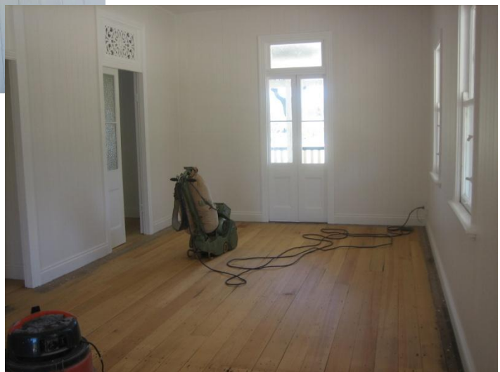
Sanding revealed the beautiful hoop pine floor boards
