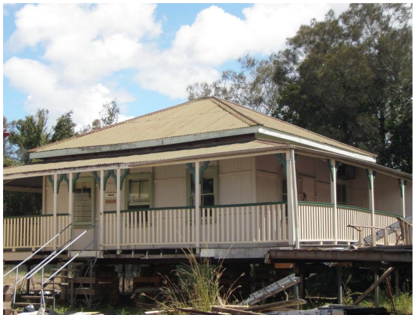
Our “orphan” – waiting to be transported to Twisted Gum Vineyard and transformed into our new cellar door
